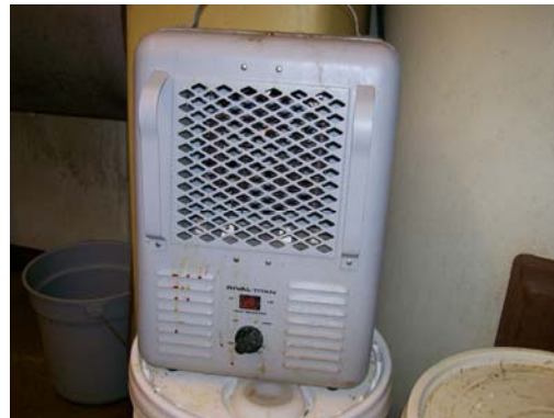
A space heater may be used during the winter in the milkhouse to keep pipes from freezing.
